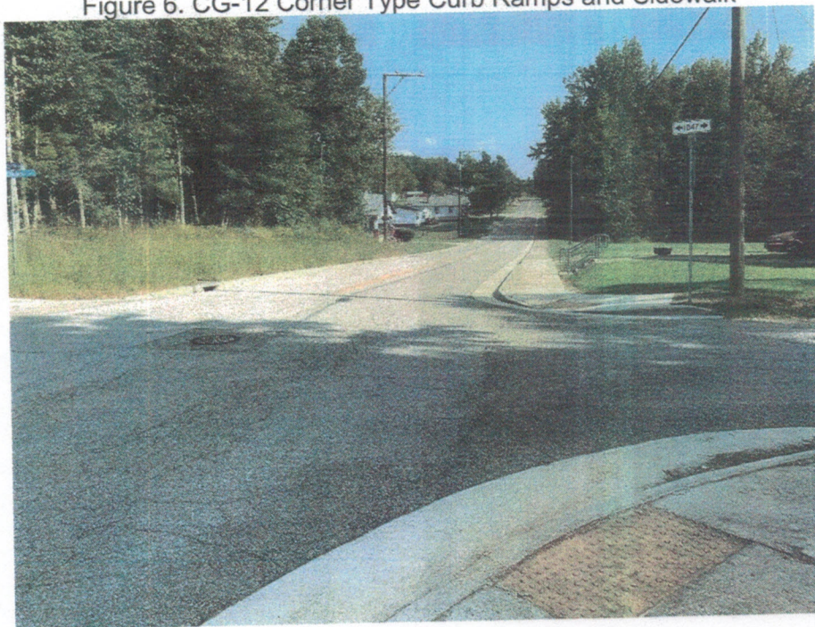
Figure 6. CG-12 Corner Type Curb Ramps and Sidewalk
